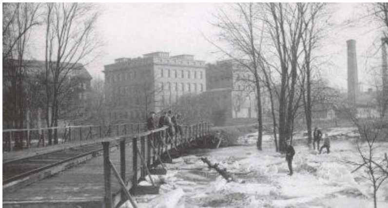
Figure 3: From Forsyth: Pere Marquette trestle over the Red Cedar River during a spring thaw, view toward the northeast, circa 1909. The square smokestack of the first boiler house may be seen at right, with second Wells Hall at left and Engineering at center. Photo Credit: M.S.U. Archives , reprinted in Nixon , p. 31.
