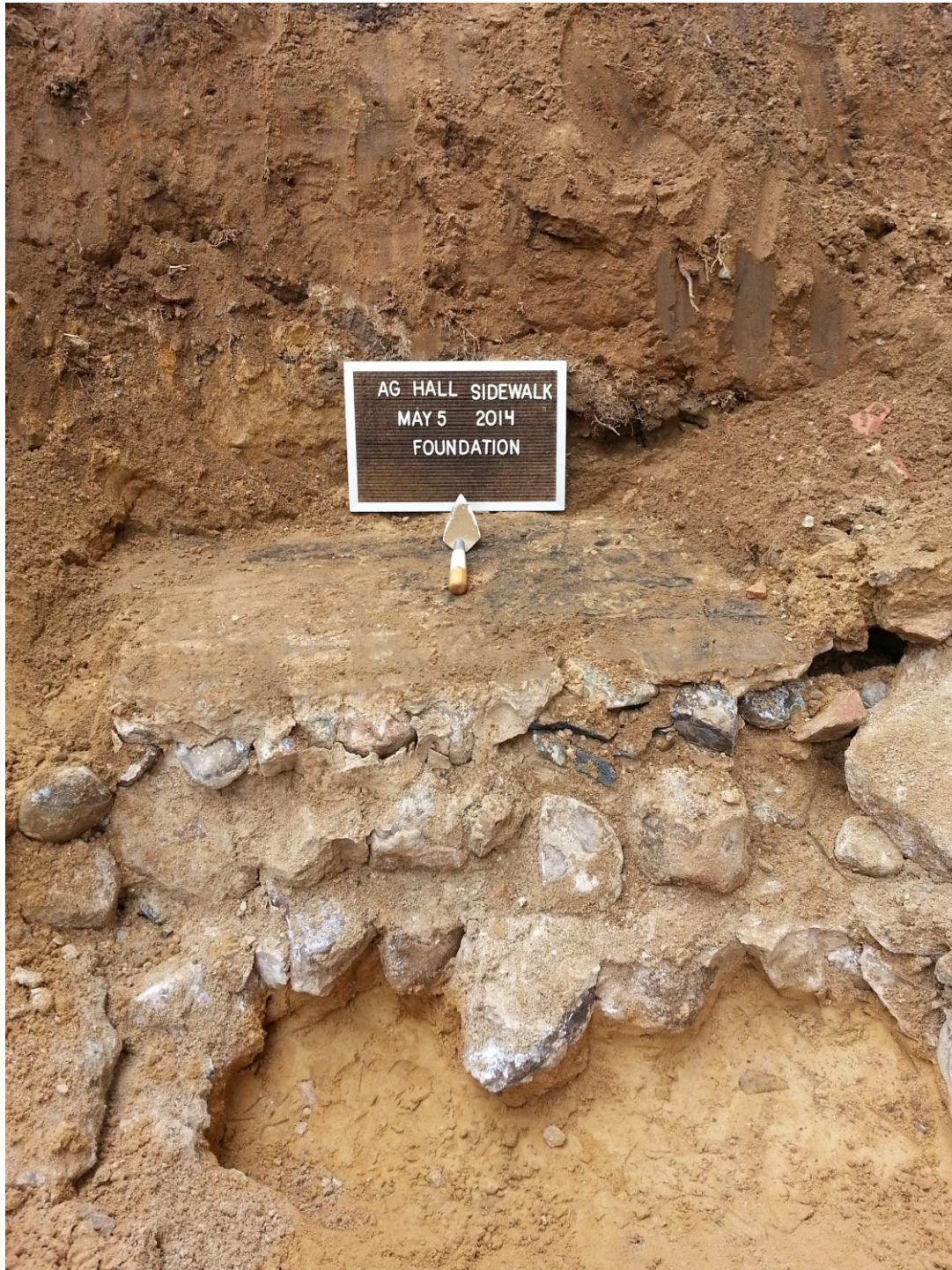
Figure 6: Photograph of feature showing courses and concrete layer
